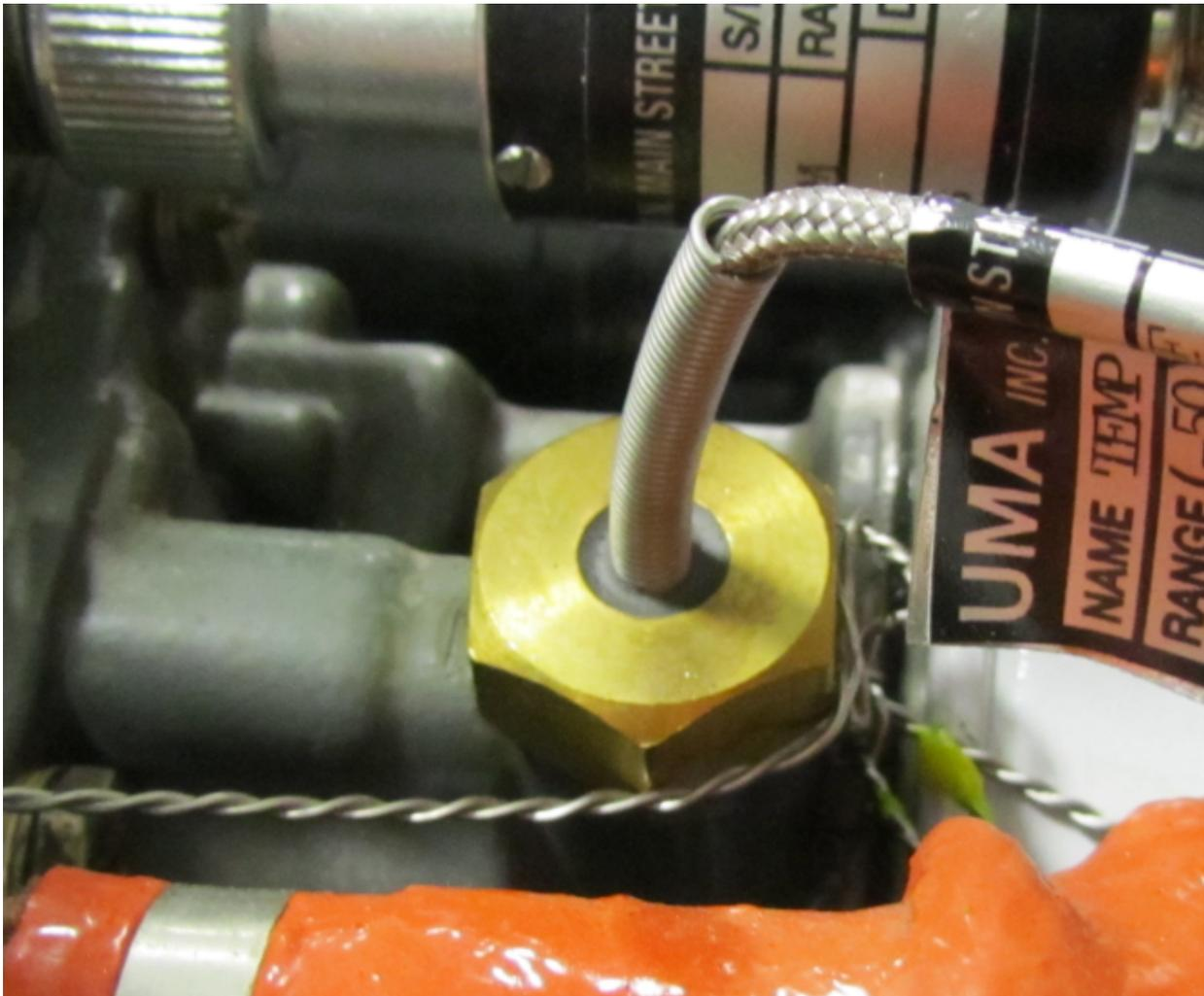
Figure 5-17 Oil Temperature Sensor Installation Example
