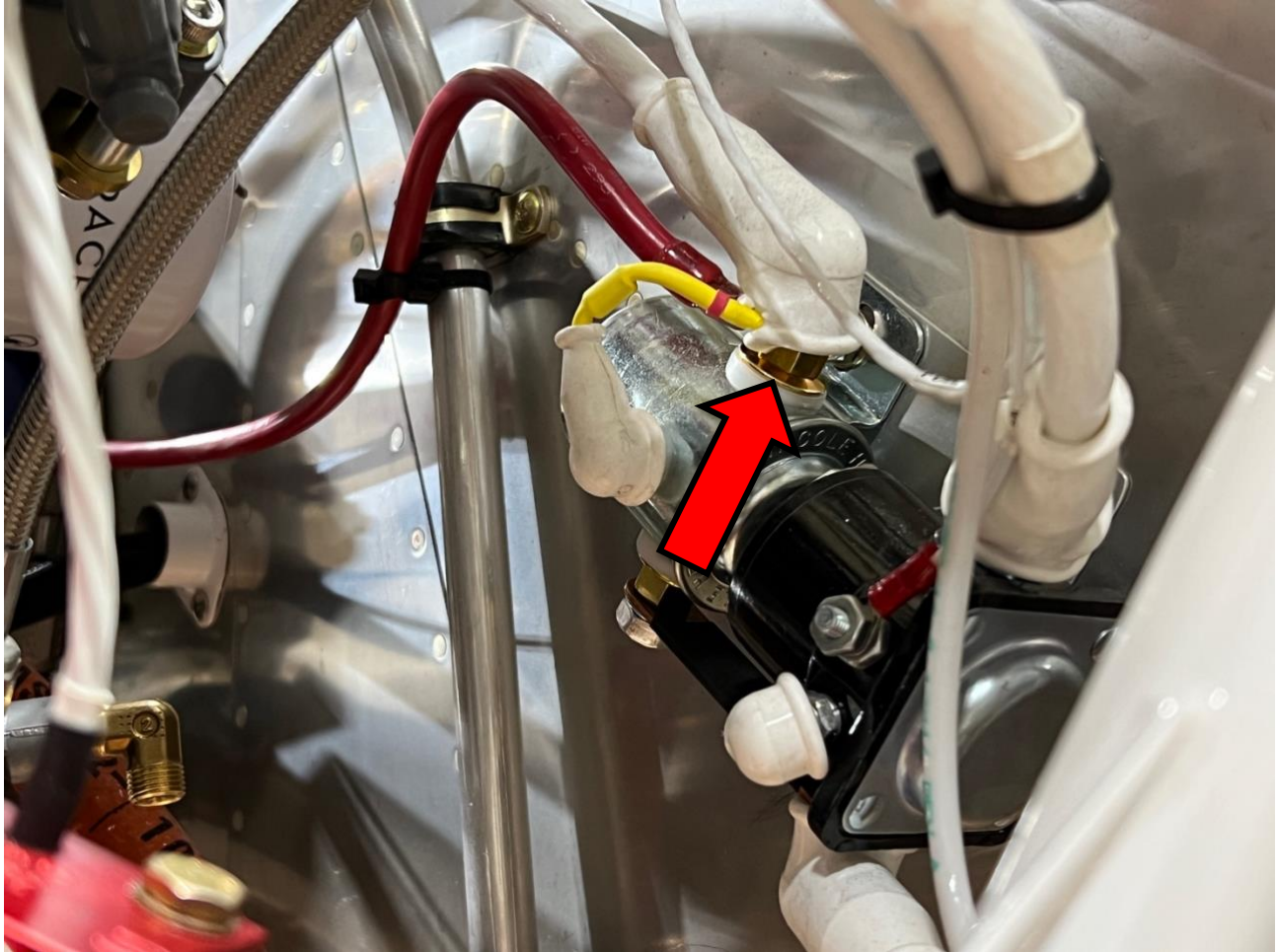
View of 2 solenoids on the left firewall - battery (silver) and starter (black). Red 6-gauge wire from external power plug is connected to the input of the battery solenoid and secured to engine breather tube to prevent vibration.
