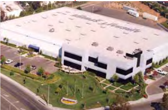
Present Home of Aircraft Spruce West (225 Airport Circle, Corona, CA.)
